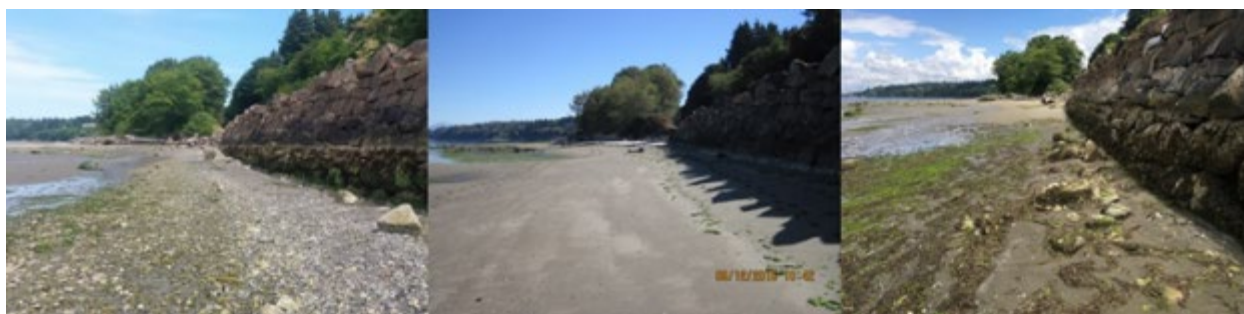
Figure 36. Site 6S/6Ar nourishment at armored location at toe of railroad - pre-project (left photo), two months post-project (center), and 35 months post project (right photo). Some drift material is still retained on the creek delta in background after 35 months.
