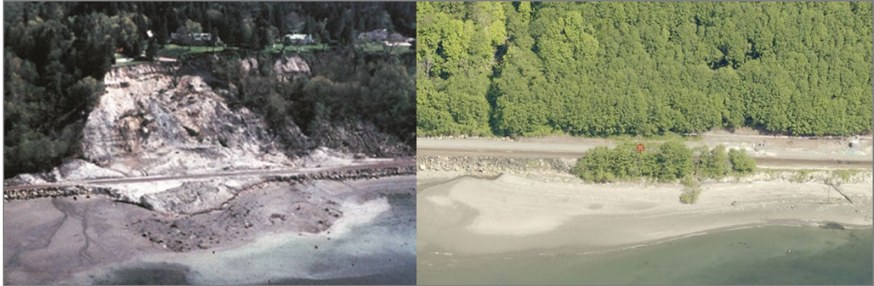
Figure 4. Oblique aerial image of deep-seated landslide at Woodway, WA (left image) taken May 1997 by E. Harp. Reprinted from USGS Bulletin 2180 (Savage et al. 2000). Woodway location in 2017 (right image), with vegetated buffer between beach and railroad. Image date 5/10/2017 from Pictometry by Eagleview.
