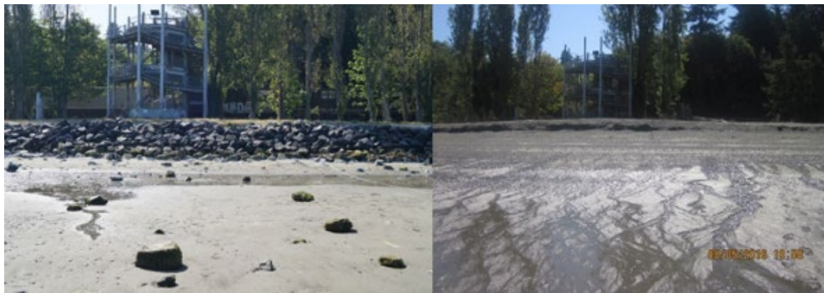
Figure 13. Howarth Park showing some of the 300 feet of shoreline armoring in 2013, and in 2016, one month post-construction. Beach access is from the pedestrian overpass in the background.
