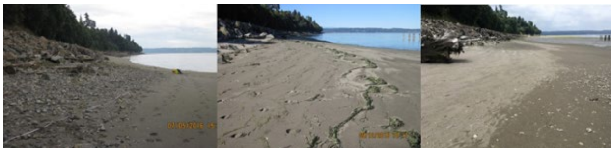
Figure 35. Site 5N at tributary delta downdrift from beach nourishment. Photos show before nourishment (left photo), with nourishment (center photo), and three years post-nourishment. Beach nourishment material is widely persistent over the area after three years.
