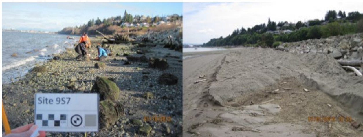
Figure 11. Site 9 beach nourishment location pre-project (left photo) and post-nourishment (right photo) still showing concentric deposits from conveyor boom prior to wave action.
