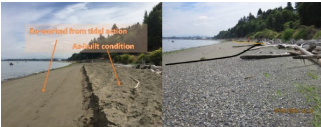
Figure 9. Site 10 as-built condition one month post beach nourishment shows concentric deposits (right side of left photo) of material placed from barge-based conveyor boom and initial drift (right photo, black line) in up-drift direction from the nourishment material (back of photo).
