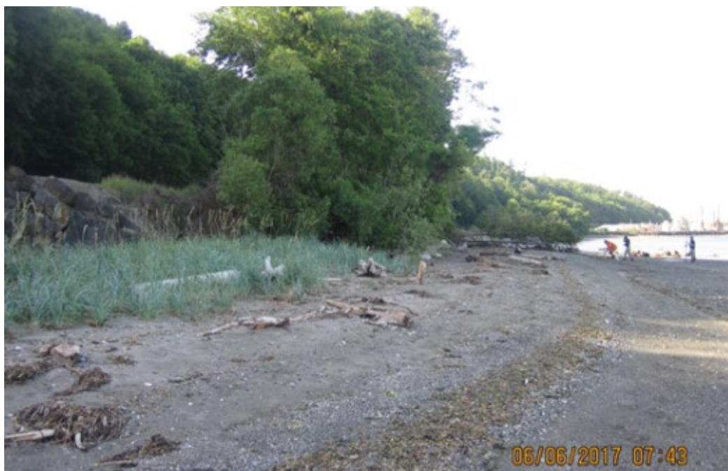
Figure 16. Deer Creek unarmored, site of the Woodway slide, 20 years post-slide. Left to right are railroad prism, back beach with dune grass, 30 cm diameter red alder trees, beach berm and log line, beach wrack, beach face, leading to beach terrace (out of photo).
