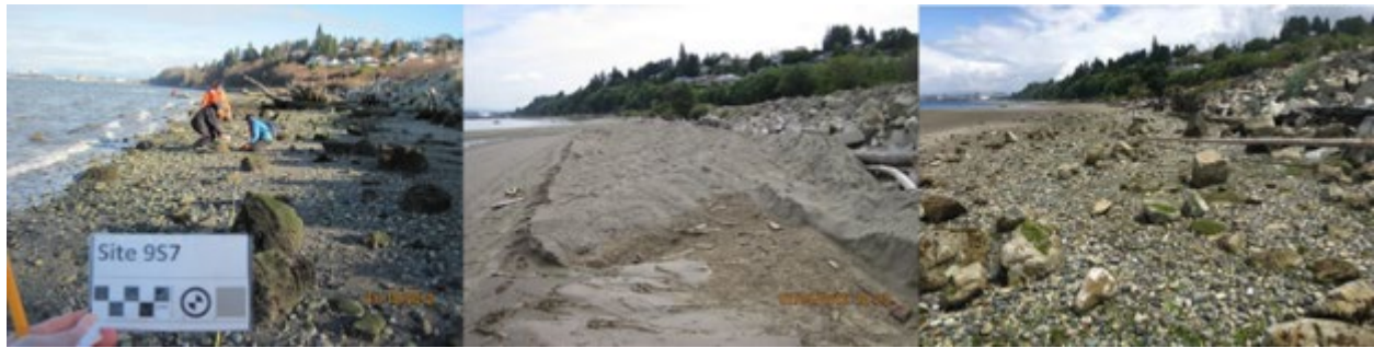
Figure 39. Site 9 beach nourishment before project implementation (left photo), beach nourishment (as-built), and in 2019, 35 months post nourishment.
