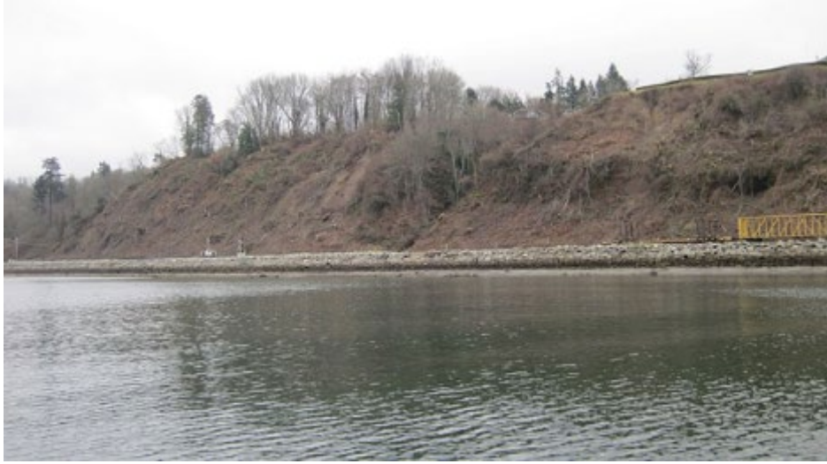
Figure 1. Typical double tracked railroad prism at shoreline of bluff-backed beach in Snohomish County
