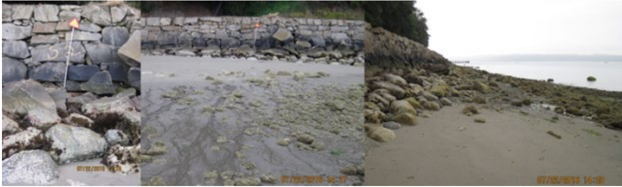
Figure 7. Site 2 shore pylon (left photo) demarcating limit of sediment placement left of pylon (center photo) and initial dispersal beach-ward (center photo) and updrift west of pylon (right photo).
