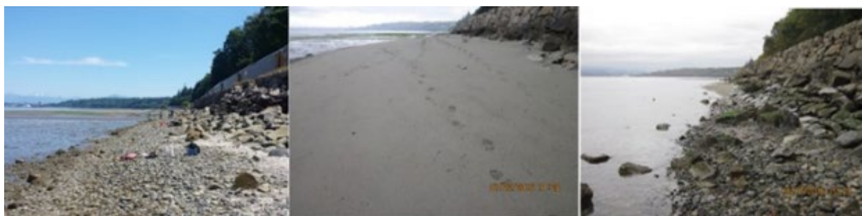
Figure 27. Site 2S Pre-project (June 2016, left), As-built (July 2016, center), and 16 months post-project (October 2017, right). Note that there is a small sand delta persistent at the back of the October 2017 photo.
