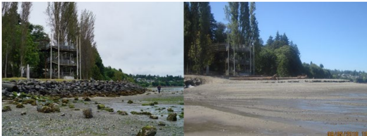
Figure 42. Howarth Park pre-project and as-built (August 2016). Riprap is removed and beach nourishment and beach wood has been placed in delta configuration as shown in Figure 13.
