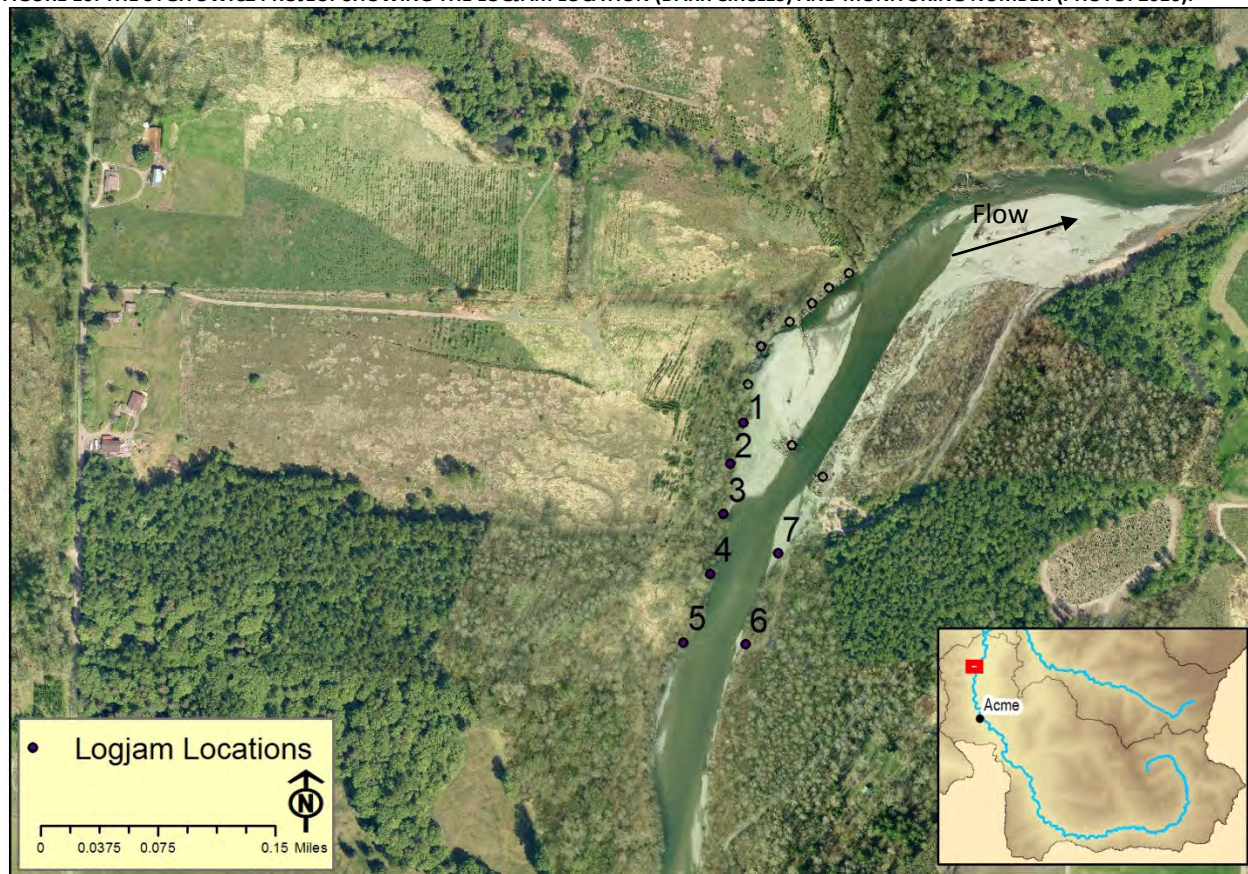
FIGURE 10: THE SYGITOWICZ PROJECT SHOWING THE LOGJAM LOCATION (DARK CIRCLES) AND MONITORING NUMBER (PHOTO: 2010).
