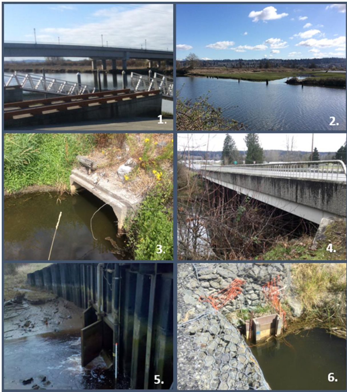
Figure B.11. Examples of the mapped water crossing feature types. 1) A channel spanning bridge classified as unrestricted. 2) A single breached levee section classified as a partial restriction. 3) A culvert classified as a significant restriction. 4) A non-channel spanning bridge classified as a partial restriction. 5) A SRT classified as a significant restriction. 6) A floodgate classified as a complete restriction.
