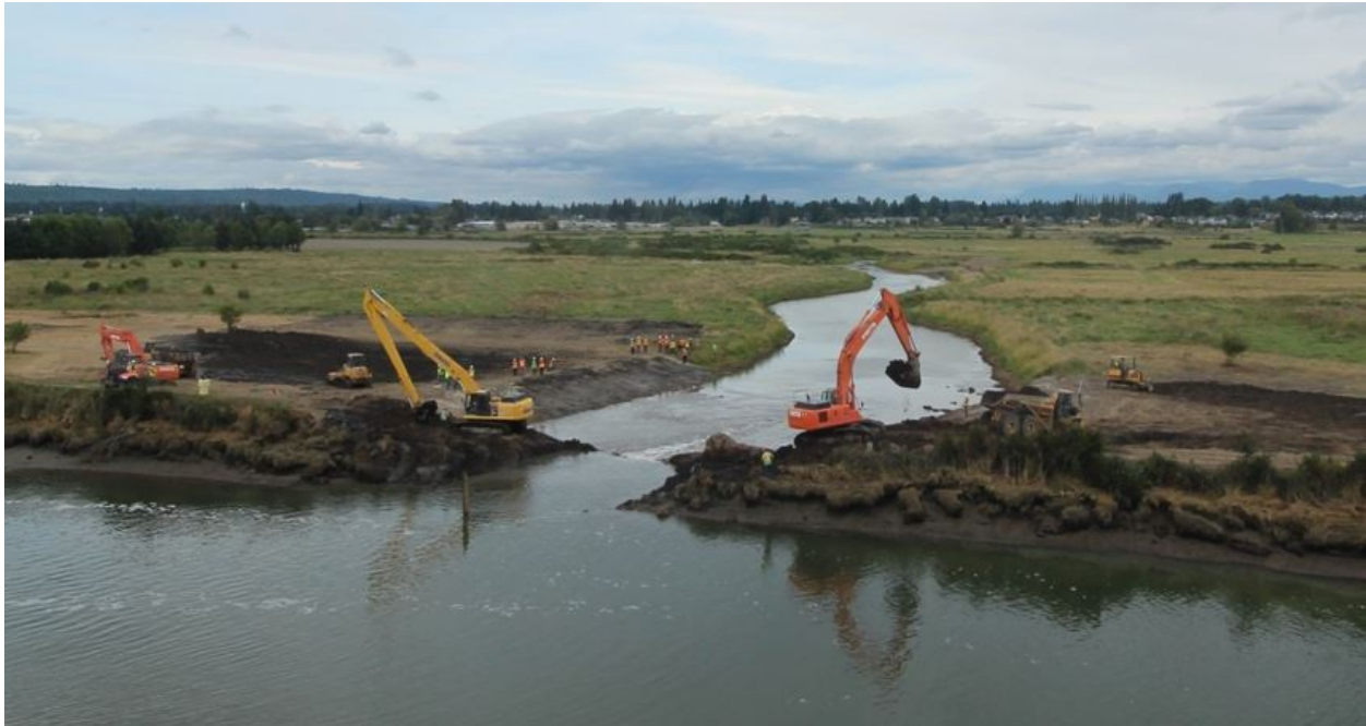
Figure 5. Photo of the final breach being cut for the Qwuloolt Estuary restoration project. This image was taken from the time lapse webcam installed at the site to provide a visual record of change over time and a public outreach tool.
