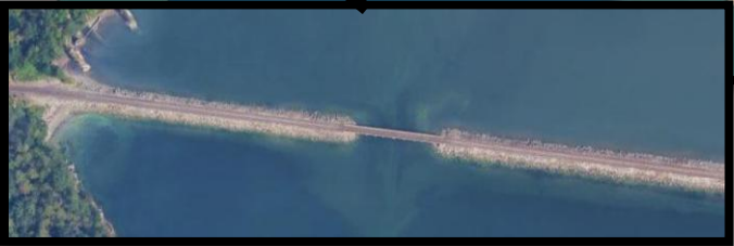
Bridge WCF classified as a Partial Restriction
