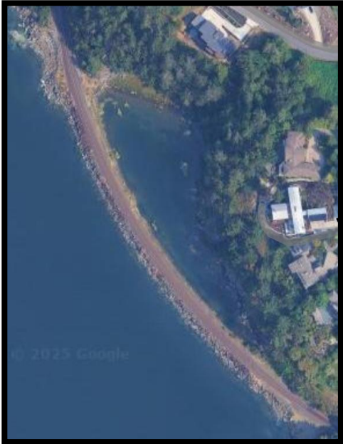
Railway without a known/visible WCF, completely disconnecting area within PMEP extent
