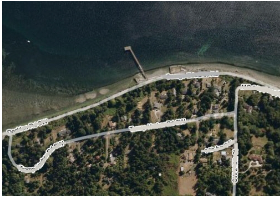
Aerial view of road area along coastline BEFORE restoration.
