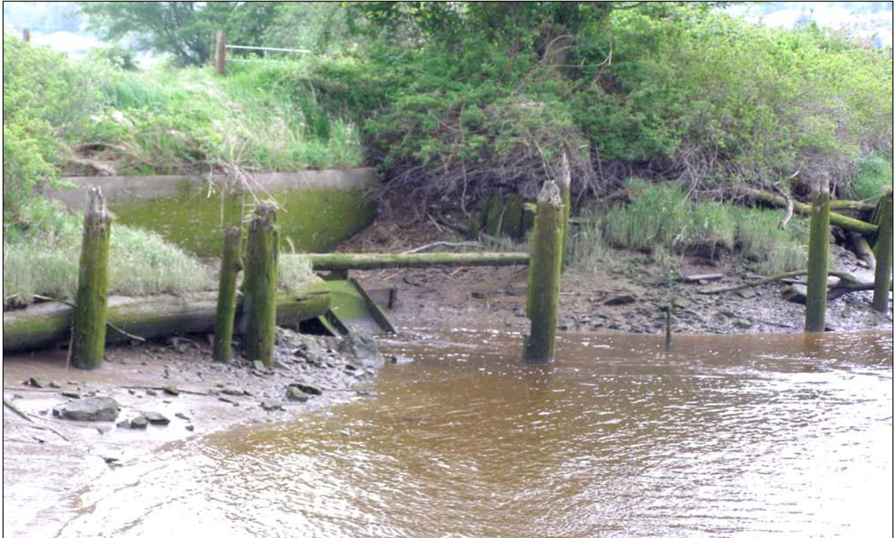
Figure 7. Tide gate outlet of Allen Creek. (photo by Zac Corum)
