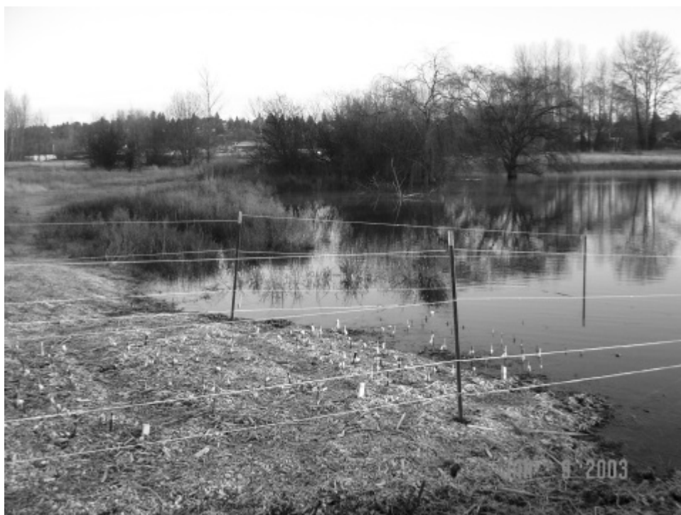
Figure B.7 – High water inundating planting block 3
