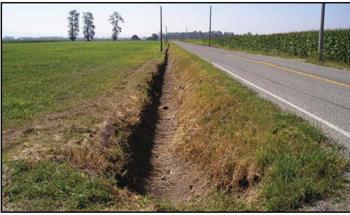
Recently maintained constructed ditch
