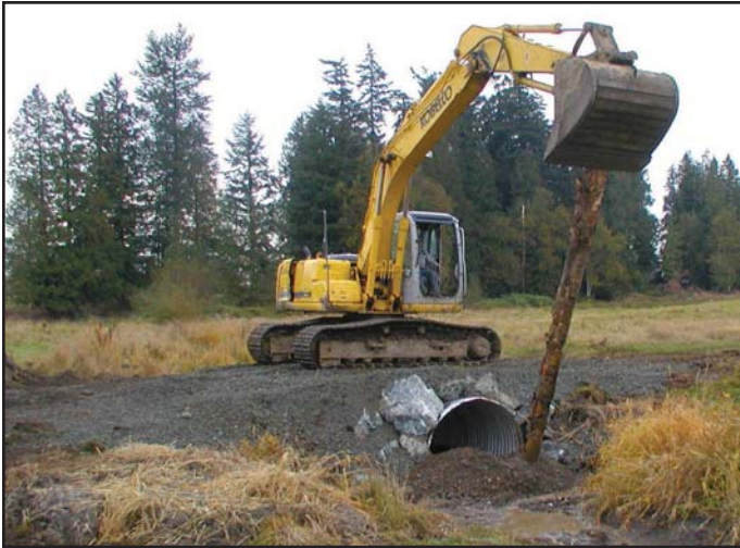
Culvert Replacement
