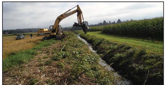
Lidded bucket on tracked excavator
