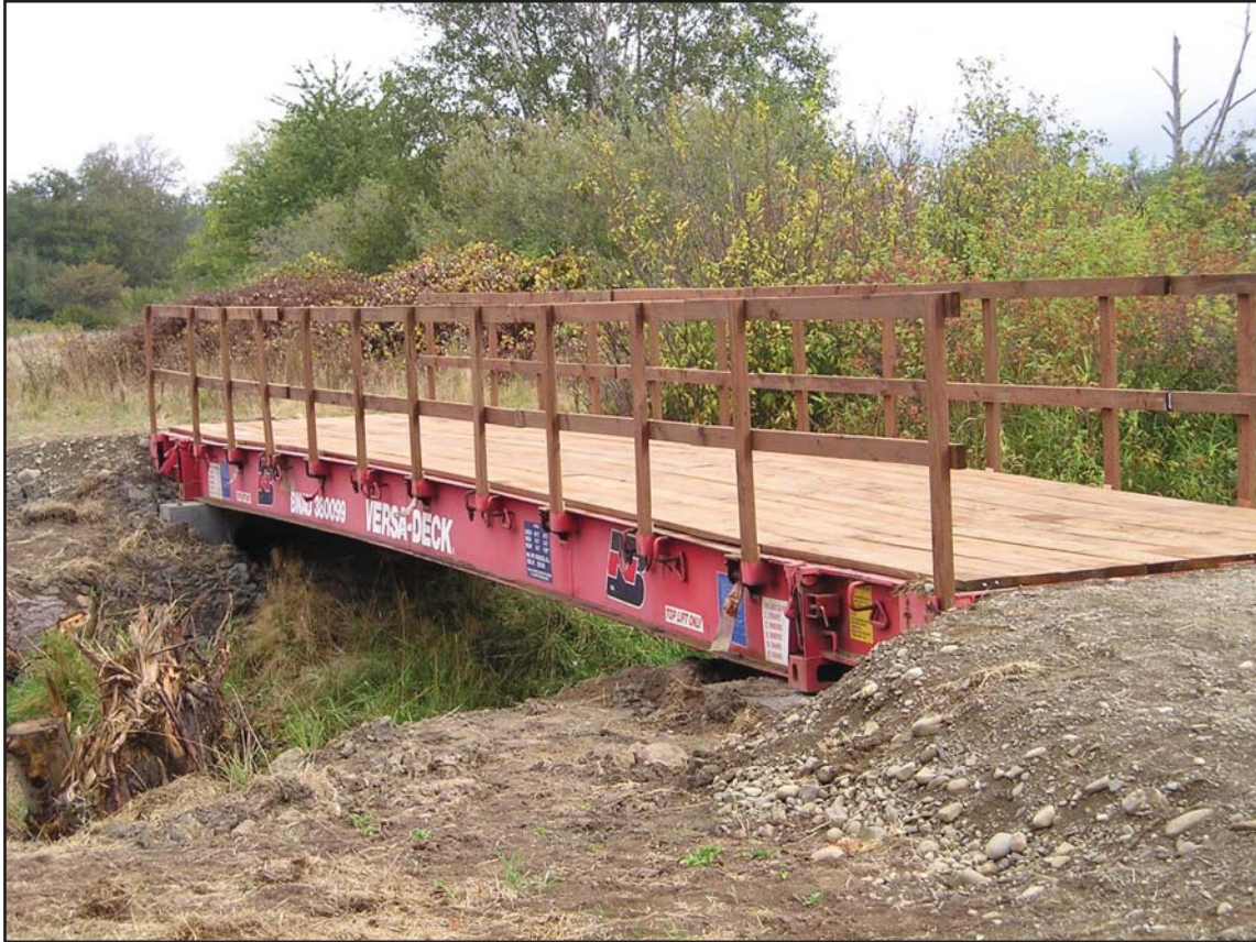
Livestock crossing made of retired rail flatcar
