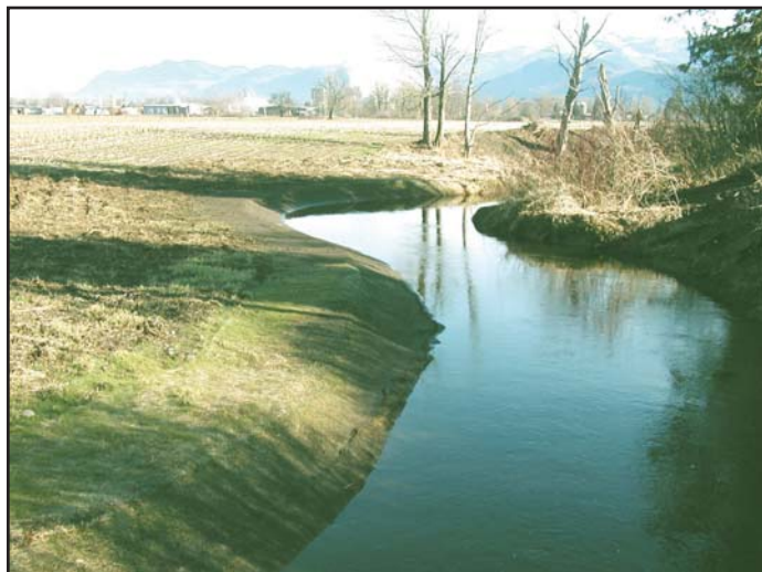
Erosion control fabric installed after maintenance work
