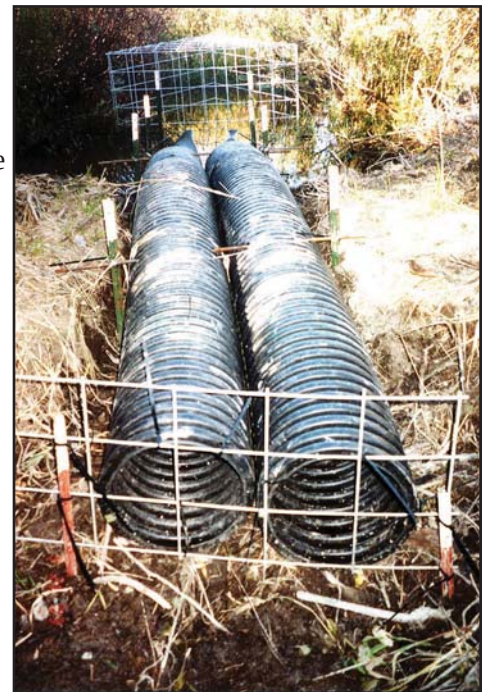
Flexible Leveler at Tennant Lake
