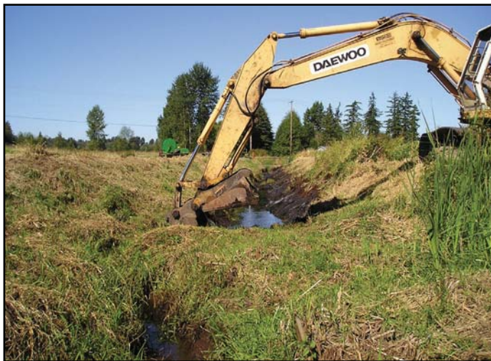
Drainage maintenance on modified natural watercourses will require a HPA
