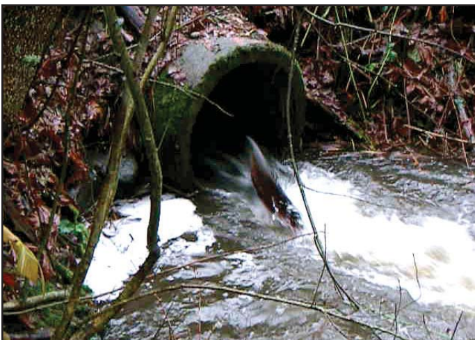
Salmon jumping at culvert.
