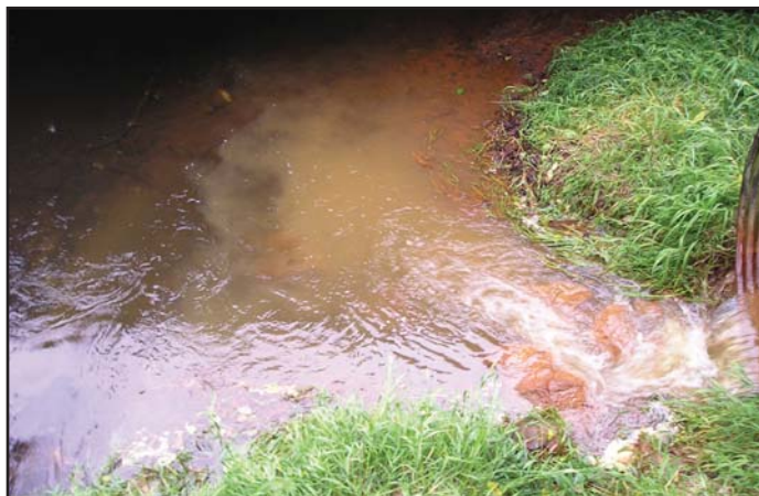
Muddy water leaving a maintained watercourse
