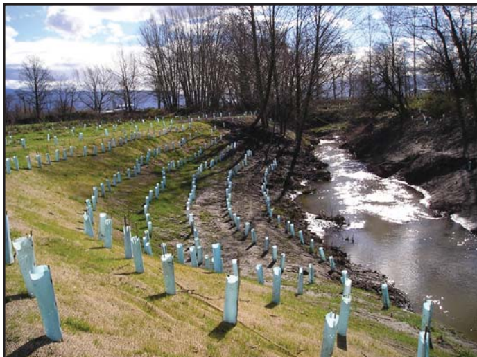
Willow livestakes planted for bank stabilization
