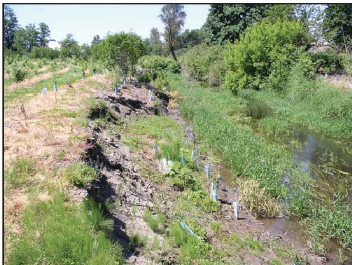
Bank failure caused by vegetation removal
