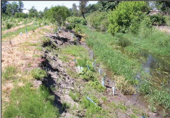
Bank Failure following herbicide application
