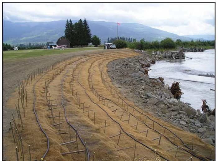
Vegetated Geogrid using Coir fabric and Willow livestakes
