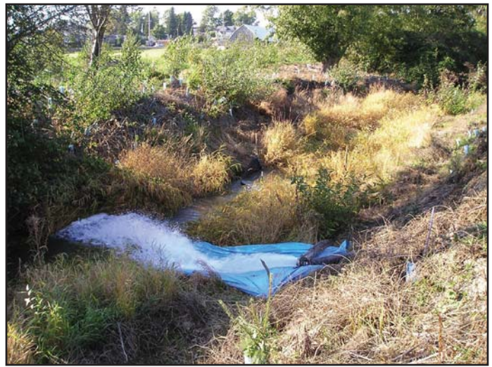
Diverted water returned to watercourse downstream
