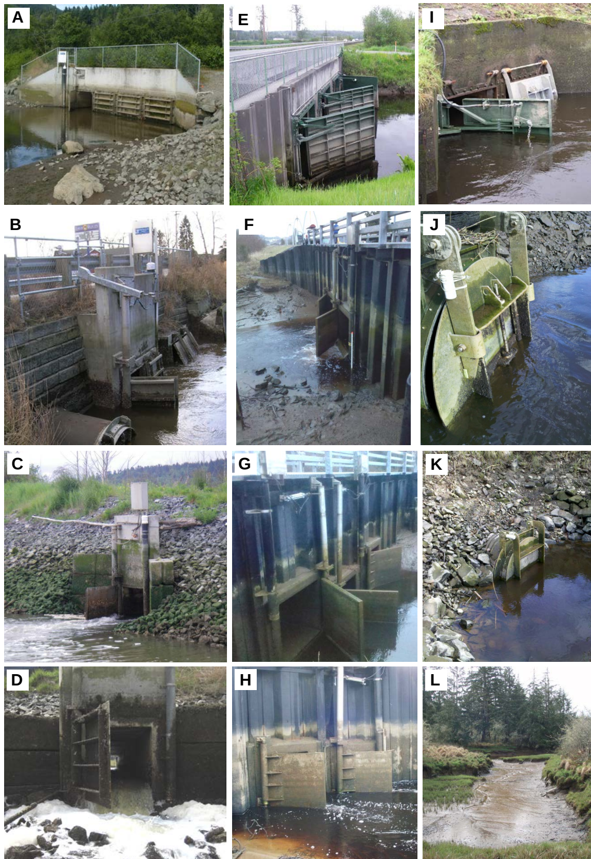
Figure 2. Self-regulating tide gates (A-J) and examples of a flap gate (K, North Hansen) and a reference site at low tide (L, Charlie Creek) used in the study design. SRTs are ordered from North to South as in Table 2. Photo credits to Jason Hall, except A (Brittany Jones), B (Oscar Bunting), C and E (Dana Rudy), D (Todd Mitchell), H (Kirsten Weinmeister), and I (Curtis Roegnor).
