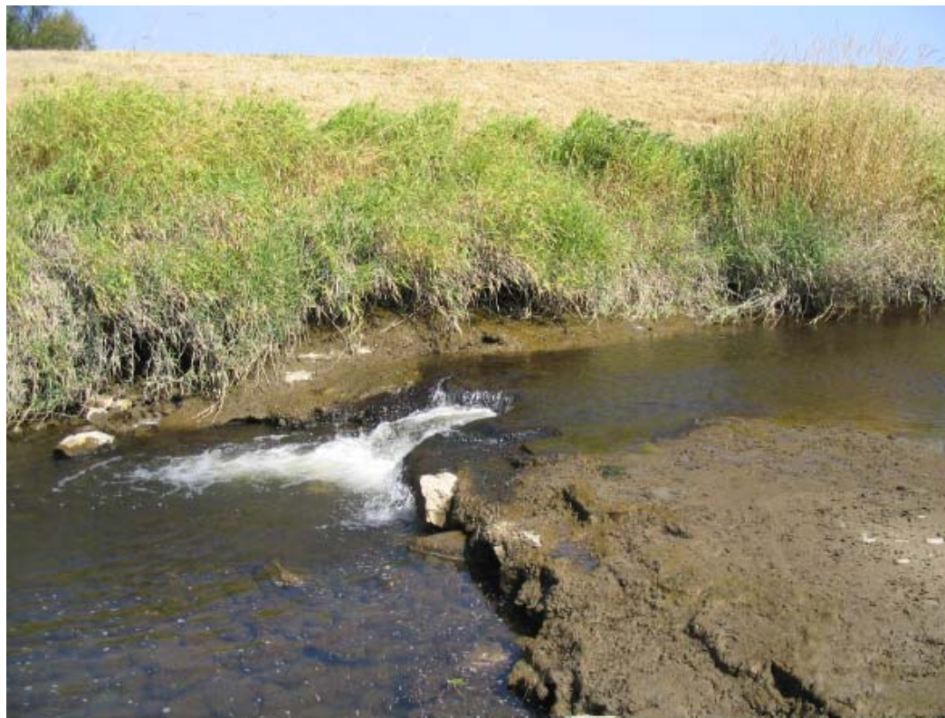
Figure 5-3. Big Ditch Structural Crown Fish Passage Barrier in Fisher Slough
