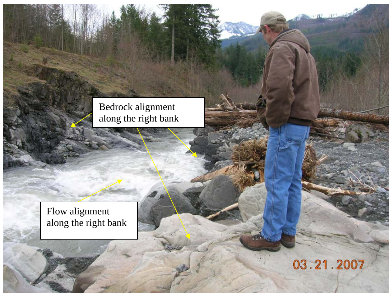
Photo 4. Segment 2 (bedrock notch) of Canyon Creek project reach, looking downstream from the right bank, March 2007. Photo by Herrera.
