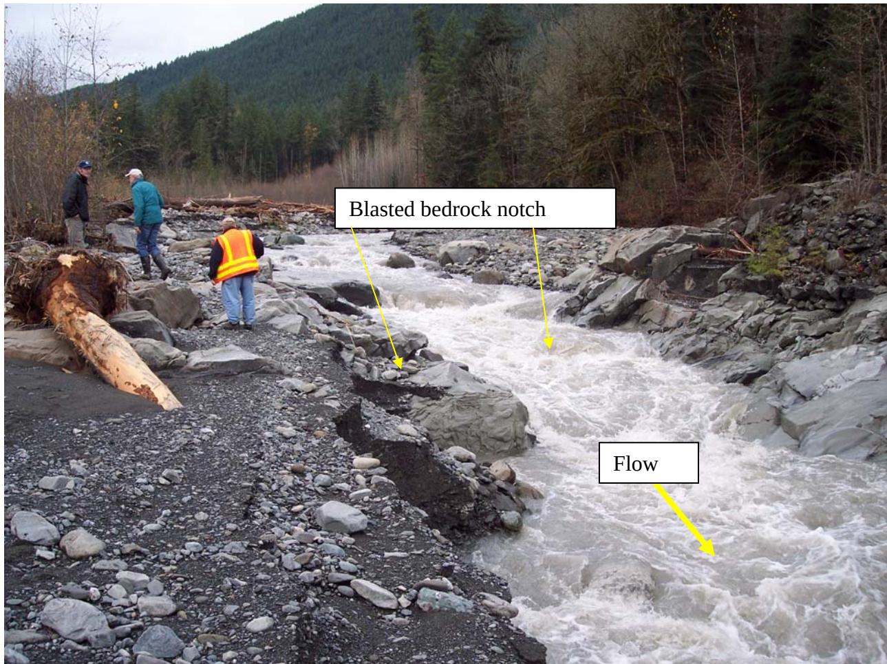
Photo 5. Segment 2 of Canyon Creek project reach, looking upstream from the right bank, February 2007. Photo by Whatcom County.
