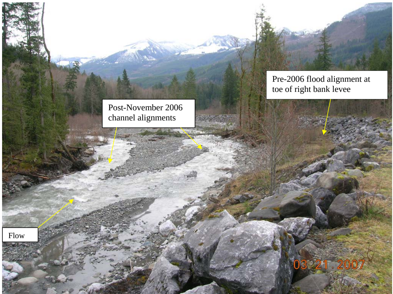
Photo 10. Segment 3 of Canyon Creek project reach, looking downstream from the right bank levee, March 2007. Photo by Herrera.
