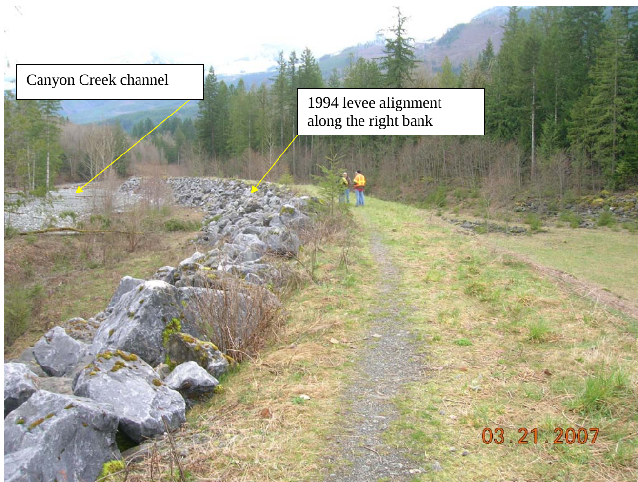
Photo 1. View looking downstream along the Canyon Creek 1994 levee, March 2007. Photo by Herrera.
