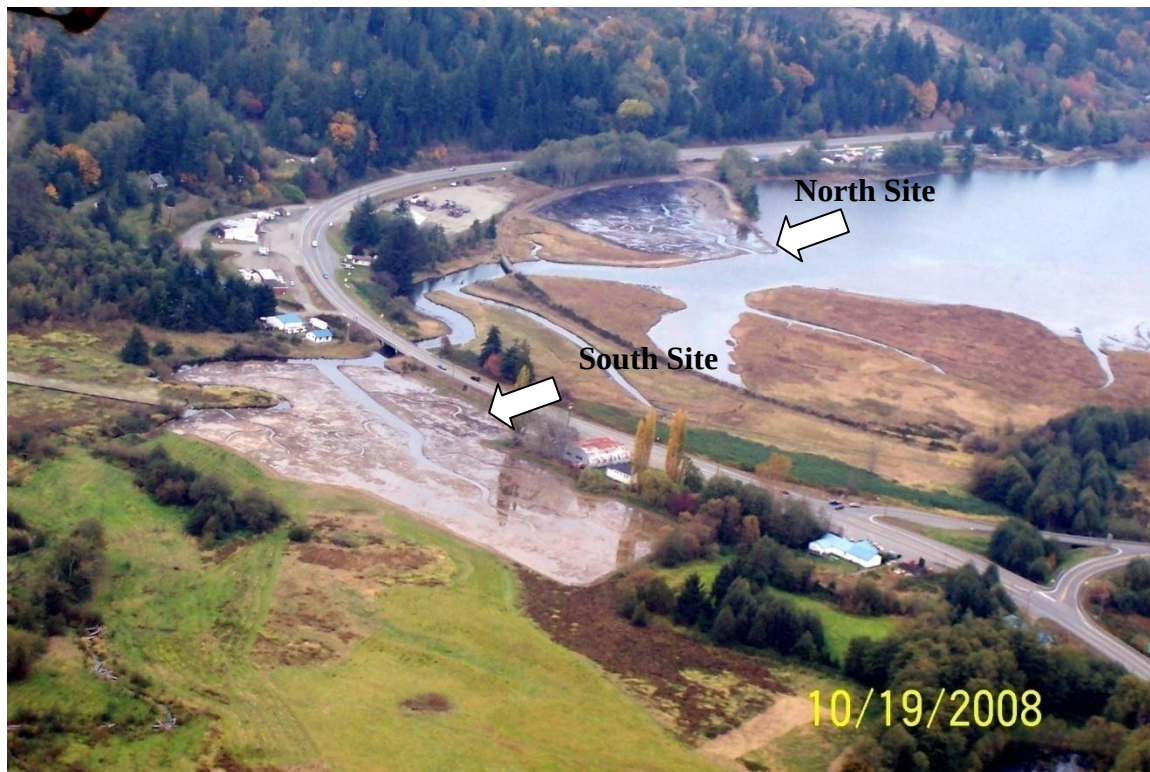
Figure 3: Aerial view from the south following construction. Note tidal channels created at south site.
