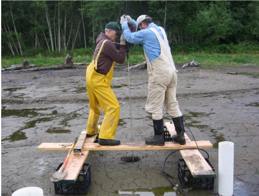
Figure 18: Sediment array during installation
