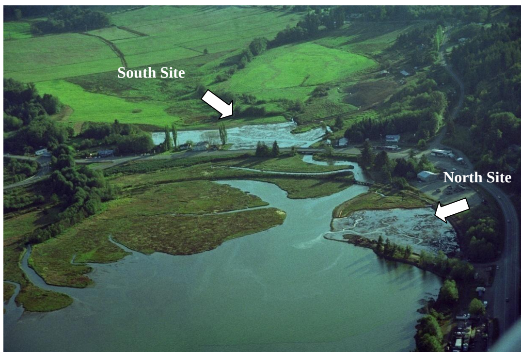
Figure 2: Project site following construction phase. Note new estuarine areas following fill removal, and tidal channel creation.
