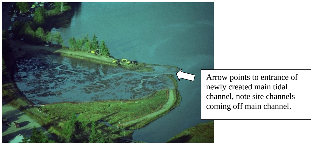
Figure 1: Tidal channels at north site, project nearing completion.
