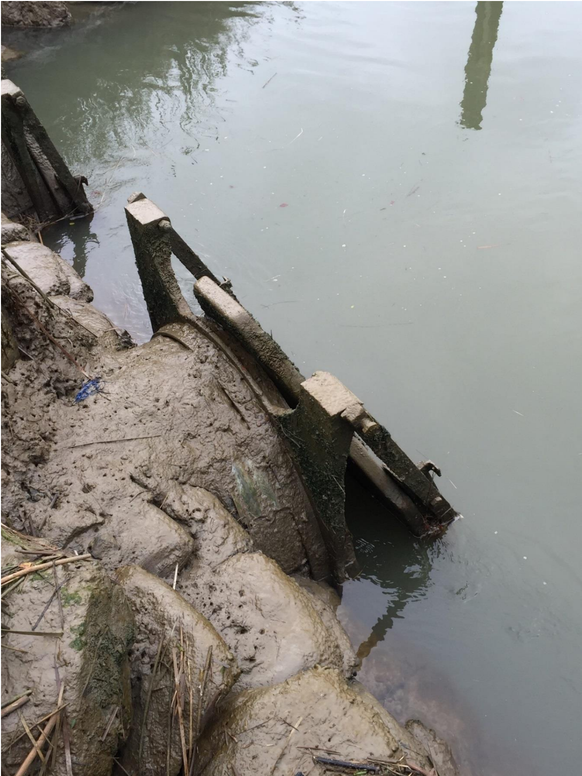
Figure 10. Fir Island Farms Tide gate open on flooding tide (October 26, 2015 at 10:40AM).
