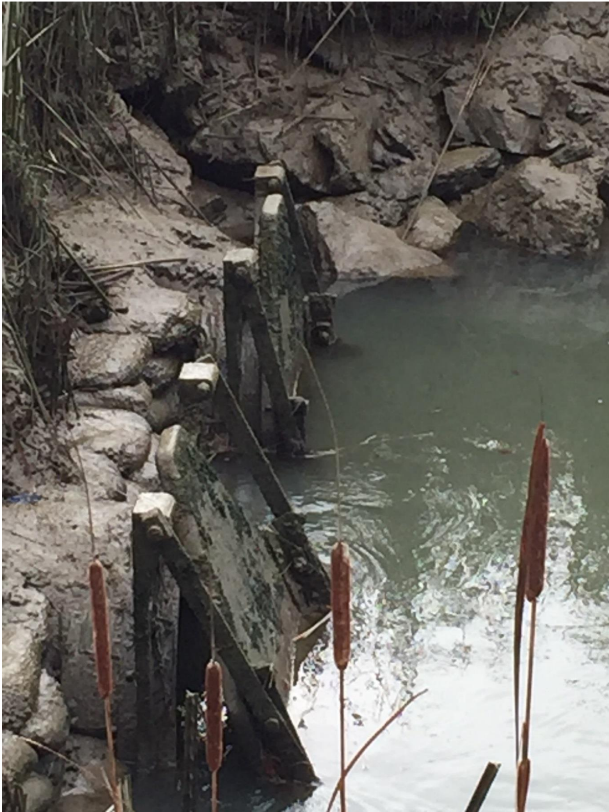
Figure 9. Fir Island Farms Tide gate open on flooding tide (October 26, 2015 at 10:40AM).
