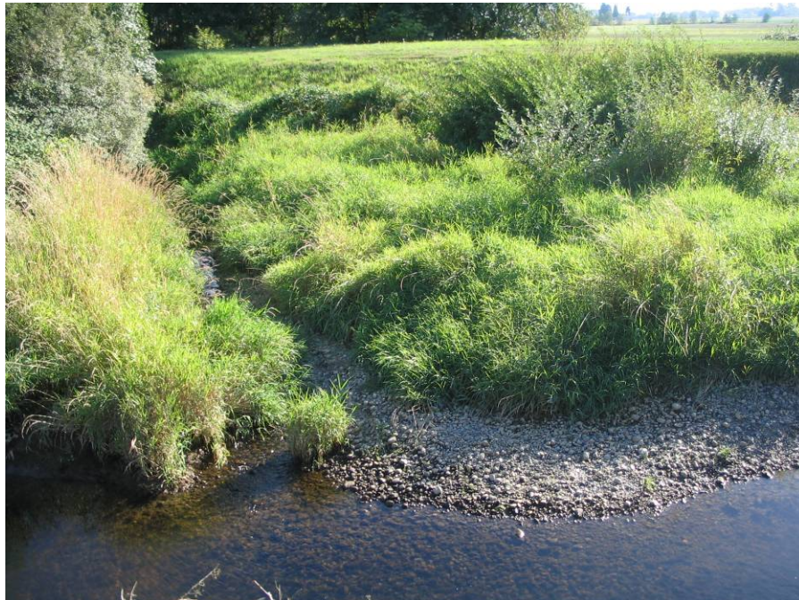
FS06-Photograph 2: Taken from the eastern end of the north levee, near an old shed and gate structure looking at Fisher Creek mouth and existing south levee. (Photo taken October 2, 2009)
