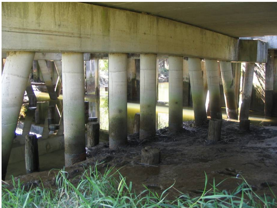
FS02-Photograph 1: Taken from the north bank of Fisher Slough at the highway bridge looking at the upstream side of floodgates. (Photo taken September 21, 2009)
