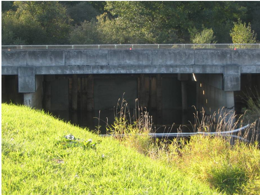
FS03-Photograph 1: Taken from the south levee of Fisher Slough looking at the upstream side of floodgates. (Photo taken September 21, 2009)
