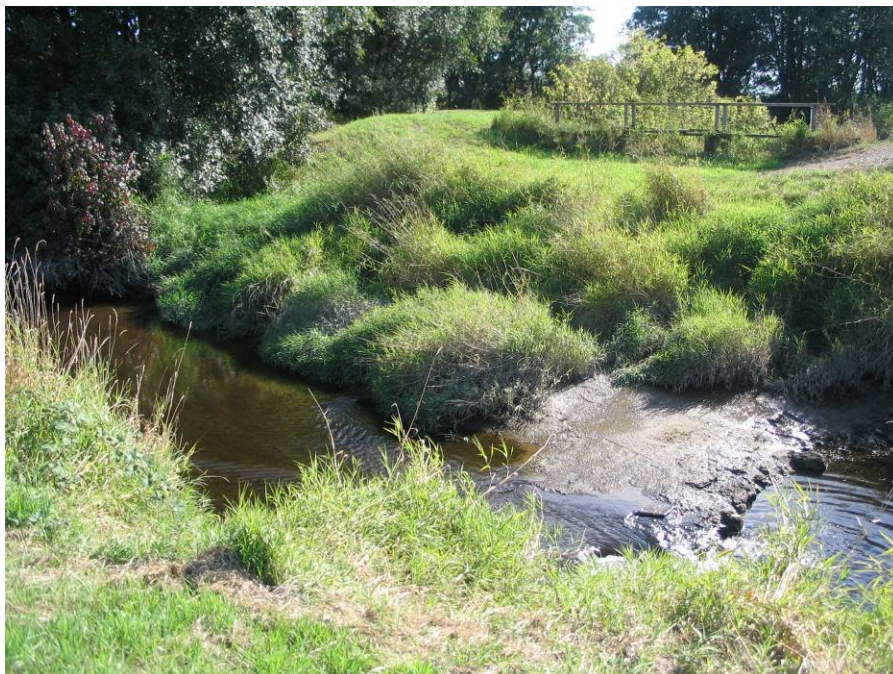
FS05-Photograph 3: Taken from the north levee of Fisher Slough at the current Big Ditch Crossing looking at the existing crossing structure. (Photo taken September 21, 2009)
