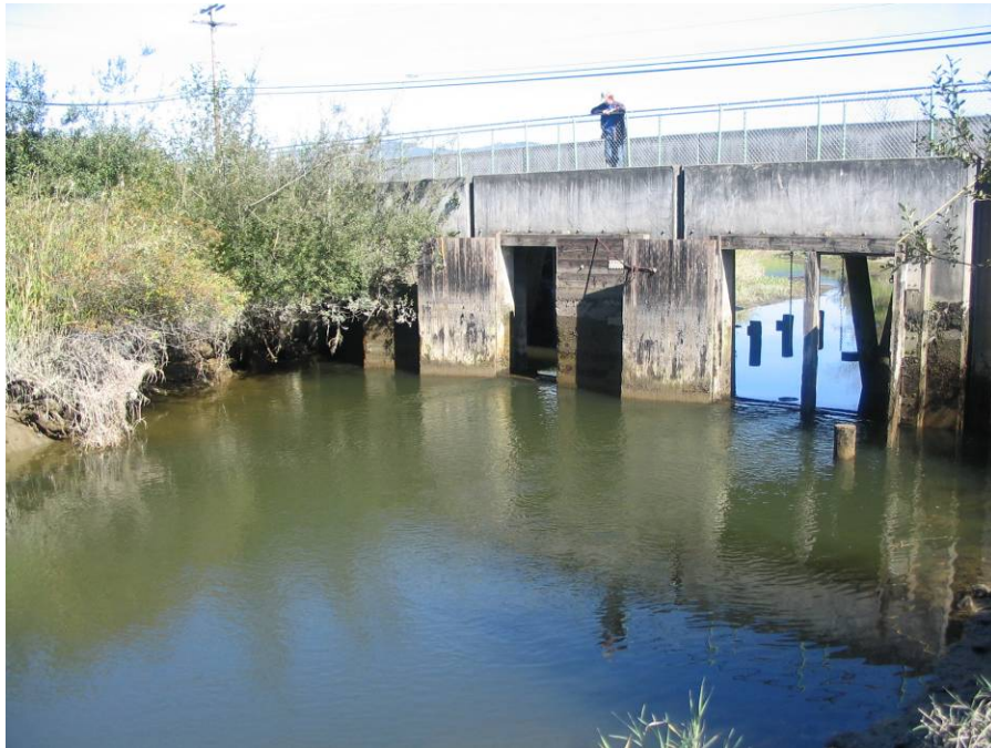
FS01-Photograph 1: Taken from the south bank of Fisher Slough at the railroad bridge looking at the downstream side of floodgates. (Photo taken September 21, 2009)
