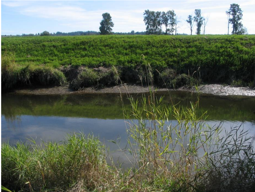
FS02-Photograph 2: Taken from the north bank of Fisher Slough at the highway bridge looking at the new crossing for Big Ditch at water level. (Photo taken September 21, 2009)
