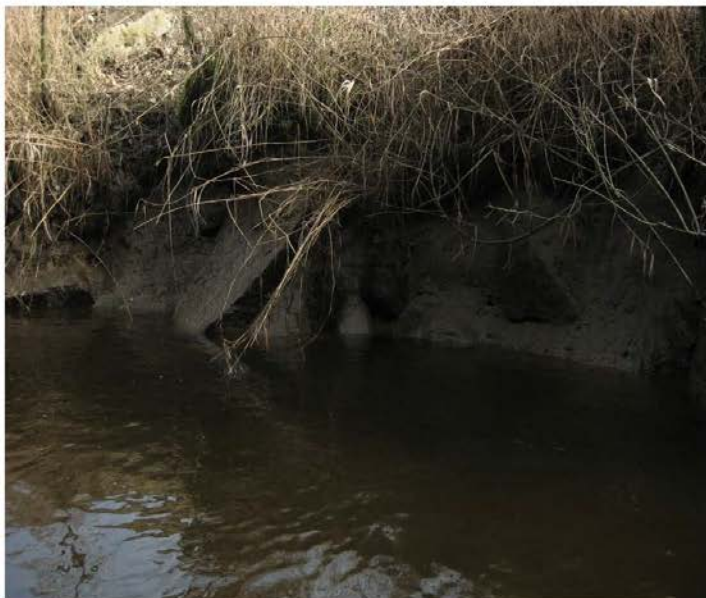
Figure 14. Looking upstream, bank protection
