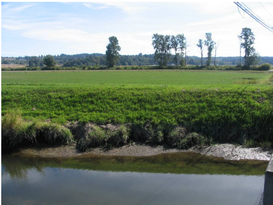
FS02-Photograph 3: Taken from the highway bridge looking at the new crossing for Big Ditch, the new south levee, and Smith A. (Photo taken September 21, 2009)
