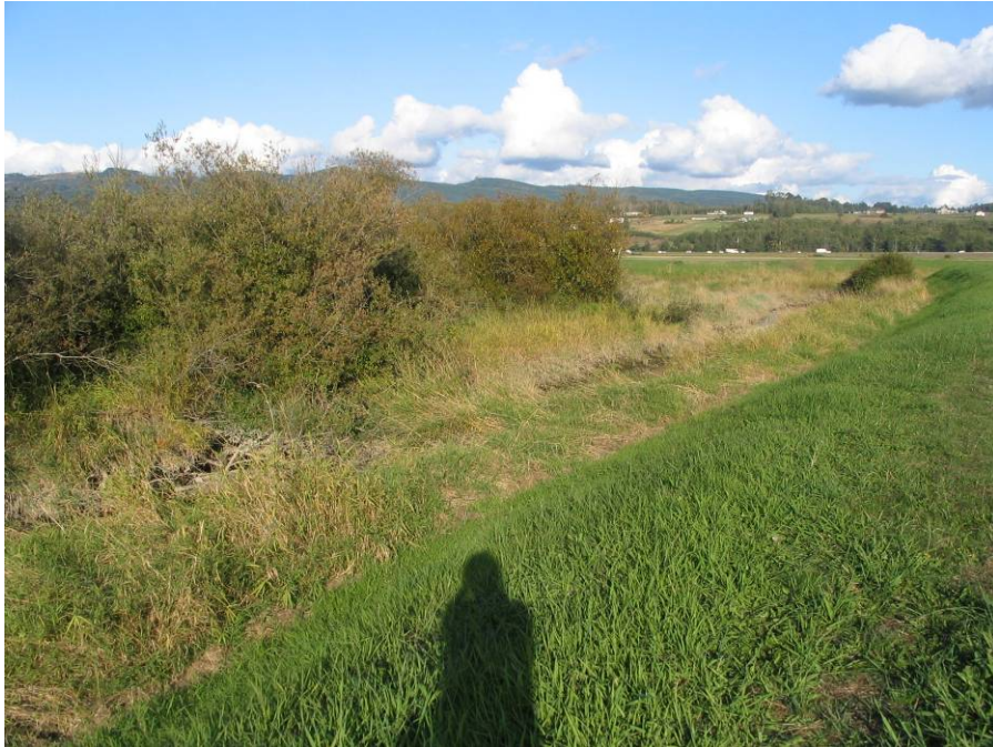
FS03-Photograph 3: Taken from the south levee of Fisher Slough looking at Fisher Slough. (Photo taken September 21, 2009)
