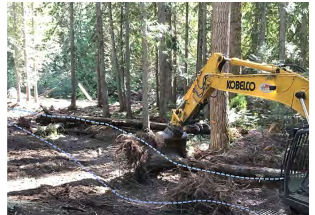
Large wood being placed to provide stabilizing roughness in a newly excavated side channel to Sullivan Creek in Pend Oreille County, WA.
