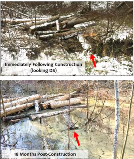
2-3 foot of channel aggradation upstream of hand-built structure in Poison Creek (Sponsor: Chelan County Natural Resource Department).
