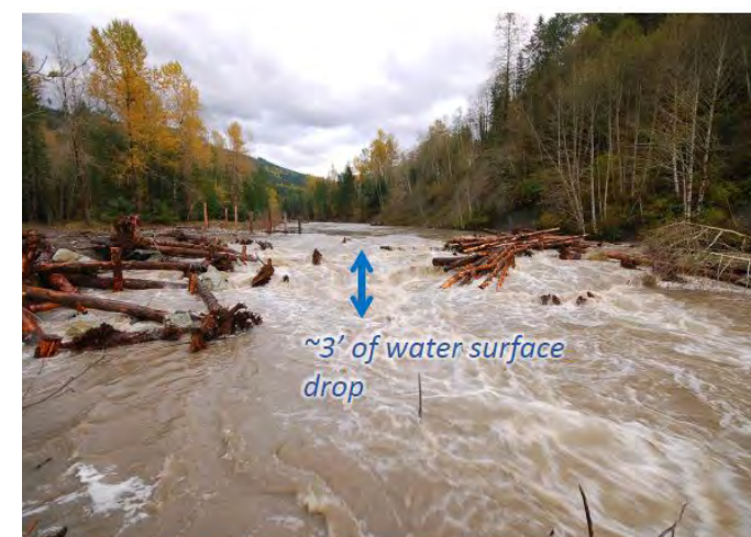
Clustered machine-built ELJs on the South Fork Nooksack River in Whatcom County, WA.
