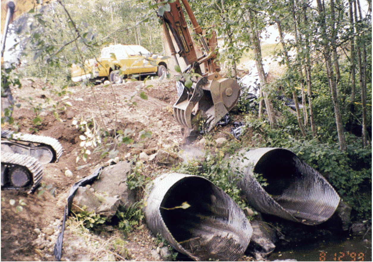
Fish Blocking Culverts Being Replaced at Simon Road
