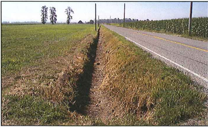
Recently maintained constructed ditch
