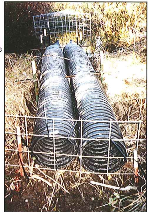
Flexible Leveler at Tennant Lake
