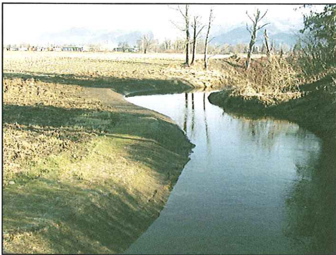
Erosion control fabric installed after maintenance work
