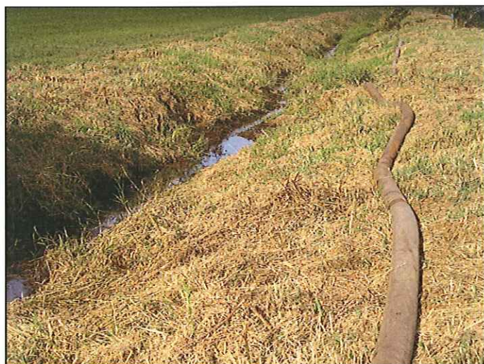
Minimal flow in work area after water is pumped around site
