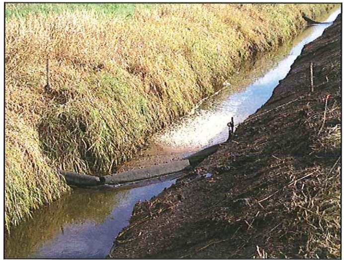
Fabric Silt Curtain slowing flow and allowing sediments to settle passes through and to slow the water flow, allowing suspended sediments to drop out.
