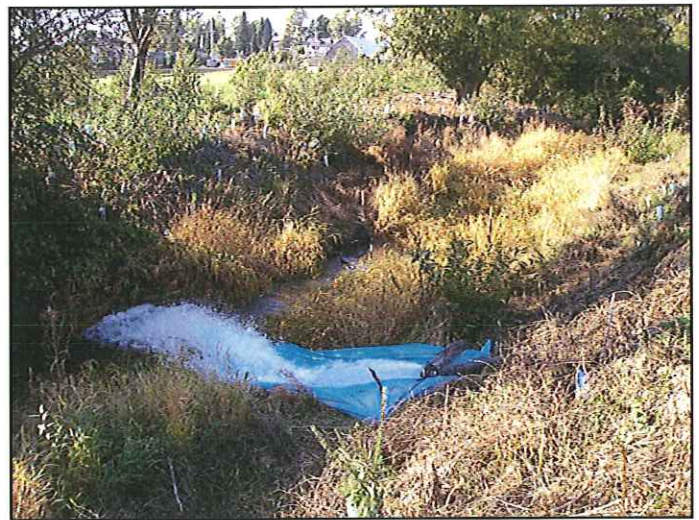
Diverted water returned to watercourse downstream
