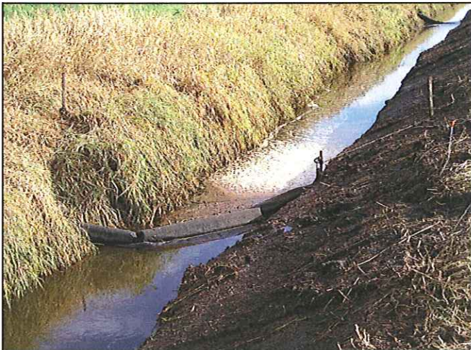
Temporary silt fence
