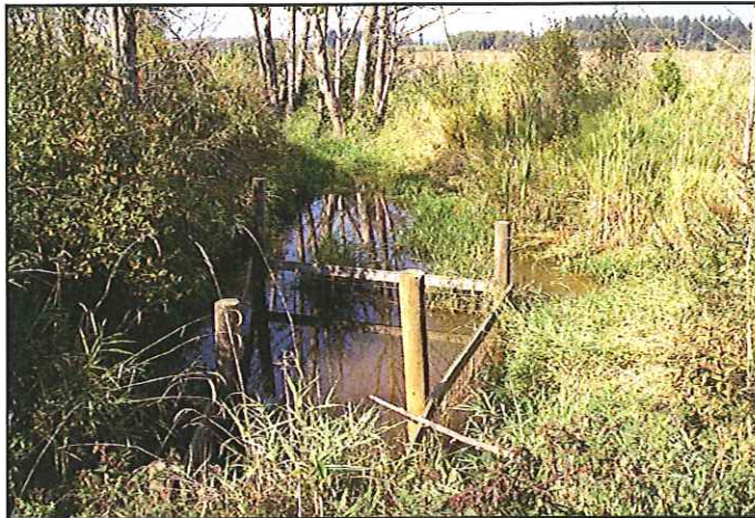
Beaver Deceiver on Schneider Ditch
