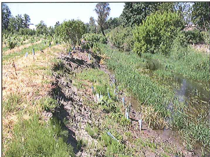
Bank failure caused by vegetation removal
