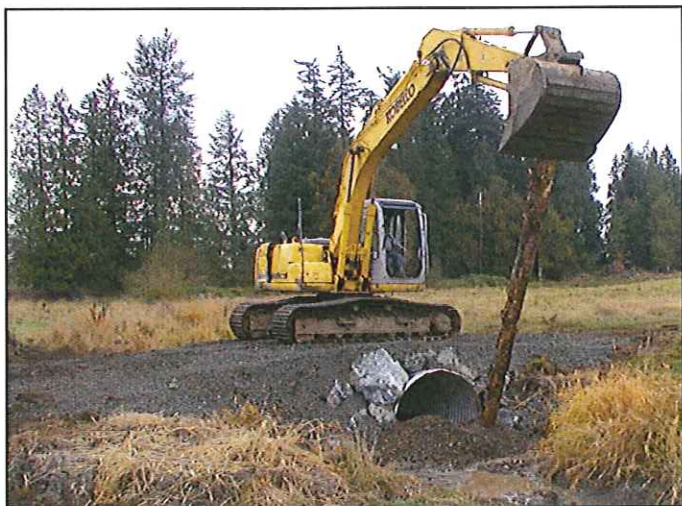
Culvert Replacement
