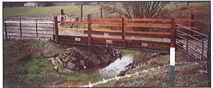
Livestock crossing made of recycled concrete bridge panels
