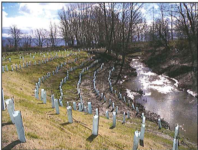
Willow livestakes planted for bank stabilization
