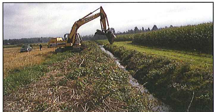
Lidded bucket on tracked excavator
