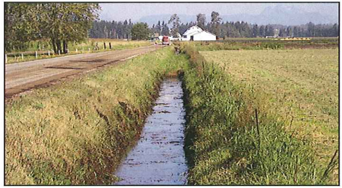
Grass strip left intact temporarily to filter sediments
