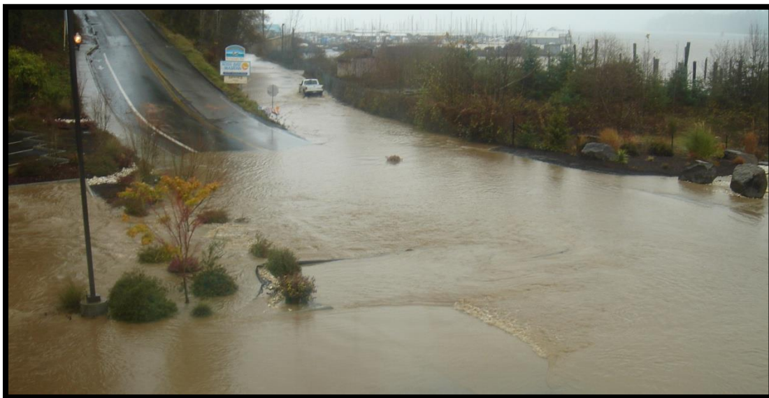
Schneider Creek Overtops West Bay Drive, December 2007
