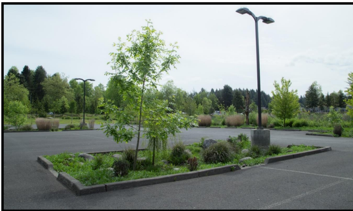
A Bioretention Cell Surrounded by Permeable Pavement, Yauger Park, 2016
