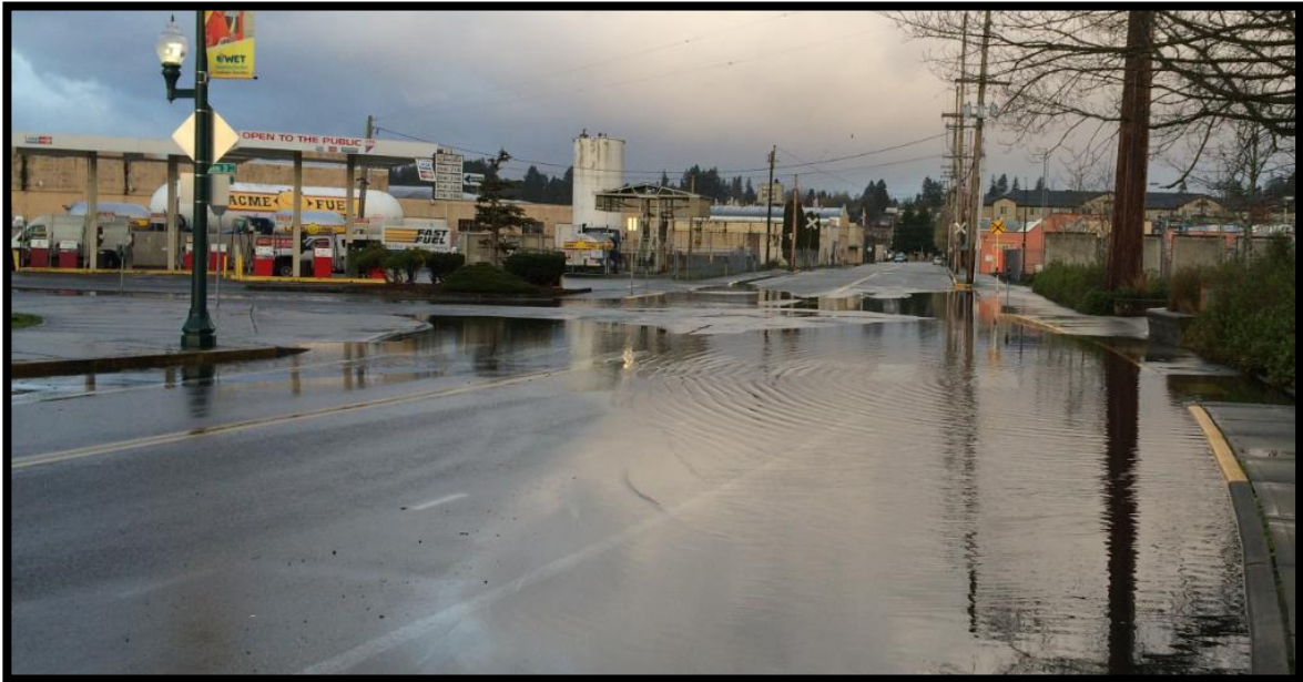
Street Flooding Due to Tidal Backflow. Thurston Avenue at Adams Street, March 2016
