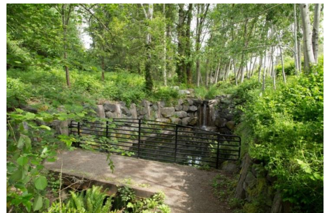
Clarification Pond at Indian Creek (May 2016)
