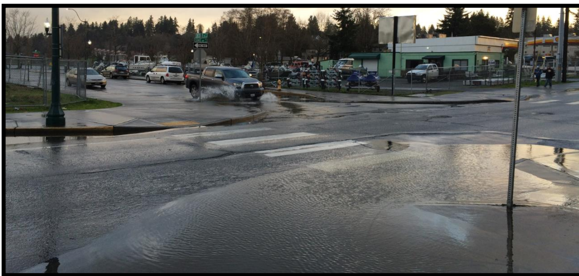
Flooding at State Avenue and Chestnut Street during High tide Following a Storm, March 2016.
