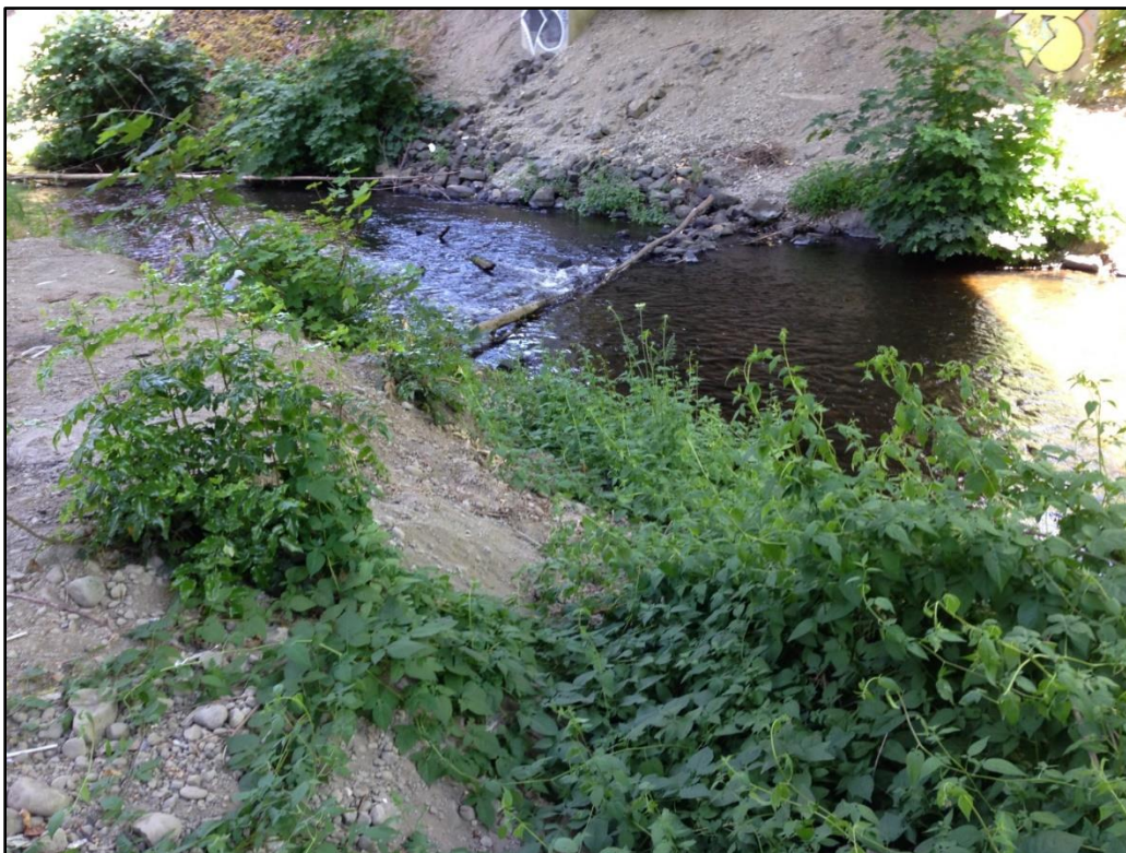
Percival Creek and Degraded Riparian Area - Under SR 101
